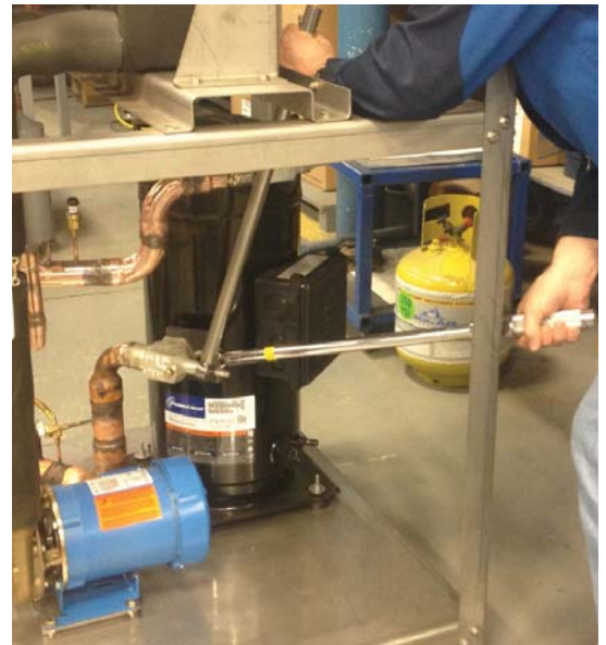
Using Colmac Crow Foot and Retaining tools to torque suction line
