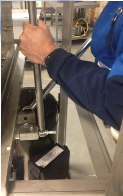
Using Colmac Crow Foot and Retaining tools to torque discharge line
