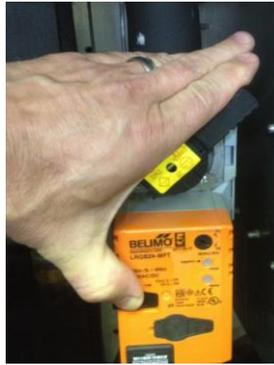
Figure 5 - Manually Moving the Lever
