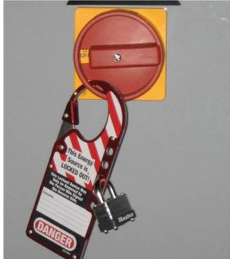
Figure 8 – Locked and Tagged Interlock
