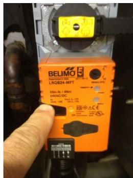
Figure 4 - Button For Manual Cycling
