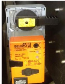
Figure 3 – e-TCV in Closed Position
