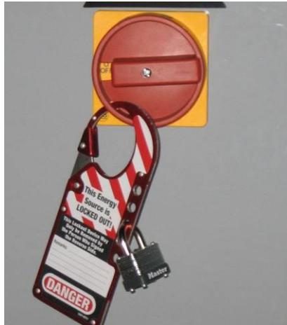
Figure 2 - Locked and Tagged Interlock
