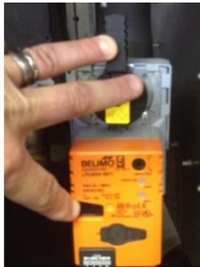
Figure 6 - e-TCV in Open Position
