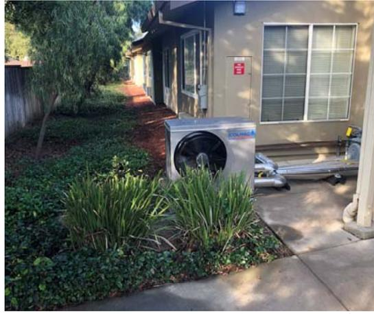
A Colmac low air source temperature CxV heat pump in California
